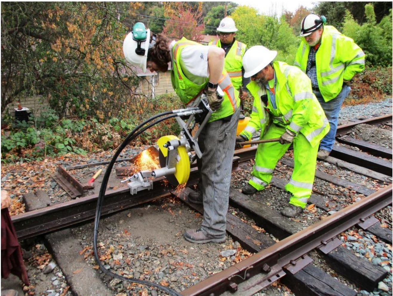
Matt cuts the rail with the new hydraulic rail-saw as Joe uses a shovel to shield the sparks
