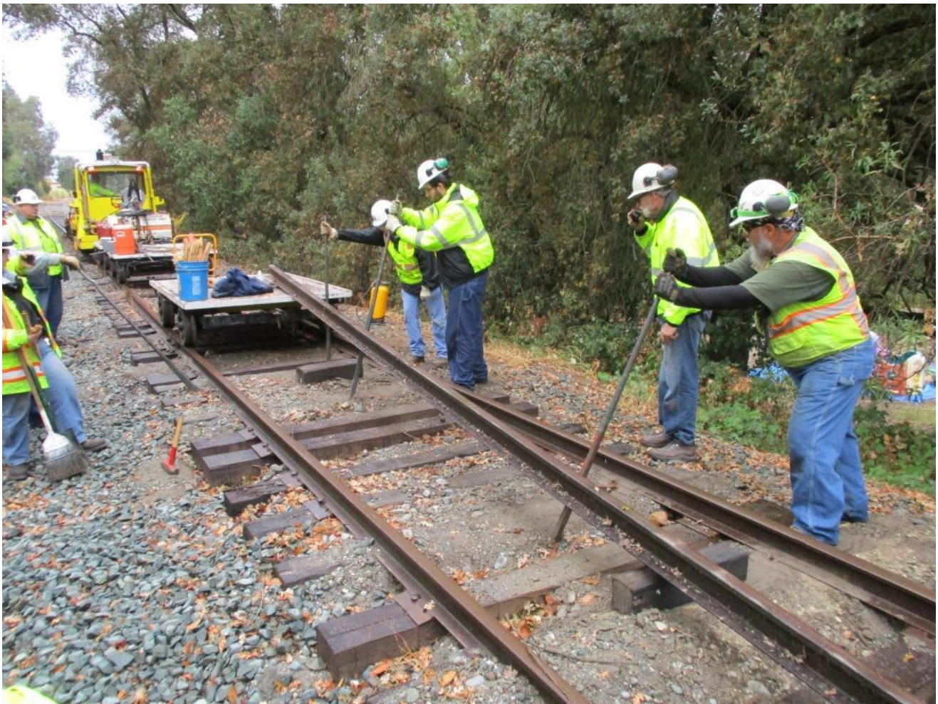
With the new rail anchored to the track, Chris C. moves the Kalamazoo south as Bill, Weston, and Mike F. use lining bars to keep it from rolling
