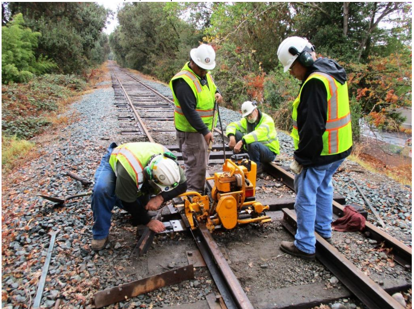
With the rail-drill clamped to the track, Anthony sprays the drill-bit with water to keep it cool while Mike F. watches for it to punch through
