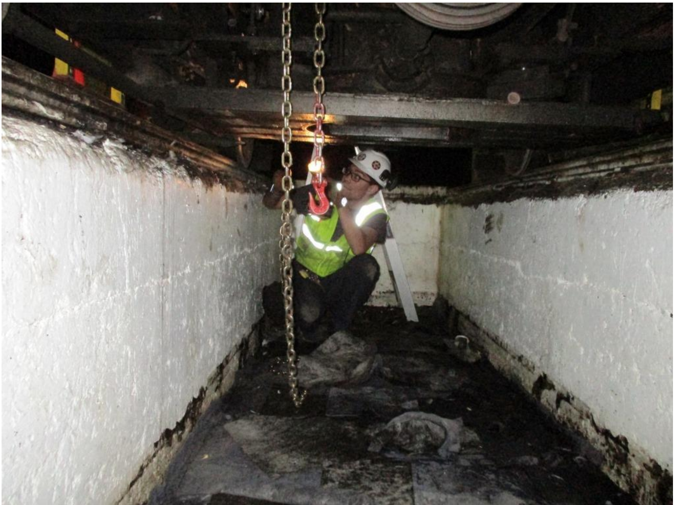
Kyle descends into the pit under the Kalamazoo to chain-up the turntable...
