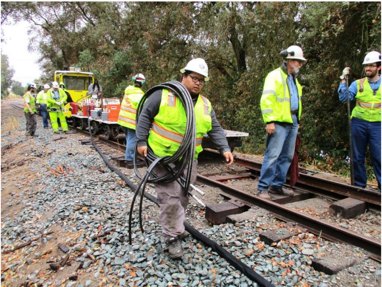
Anthony deploys the hydraulic hoses for use by the new hydraulic rail-saw
