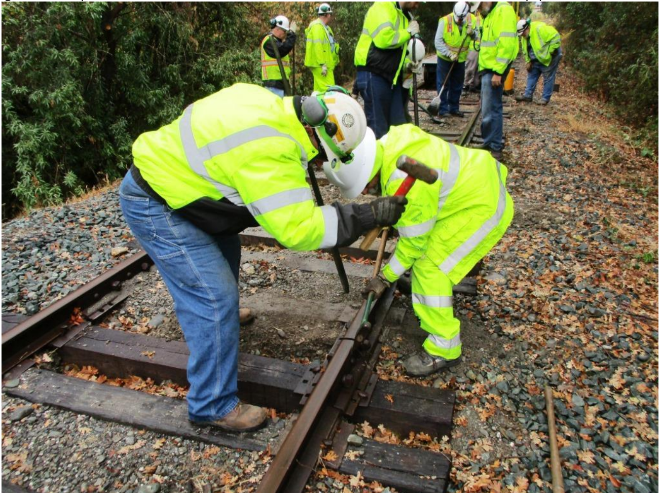
Joe holds the chisel as Mike F. unleashes the hammer on it to break the bond-wire off the track
