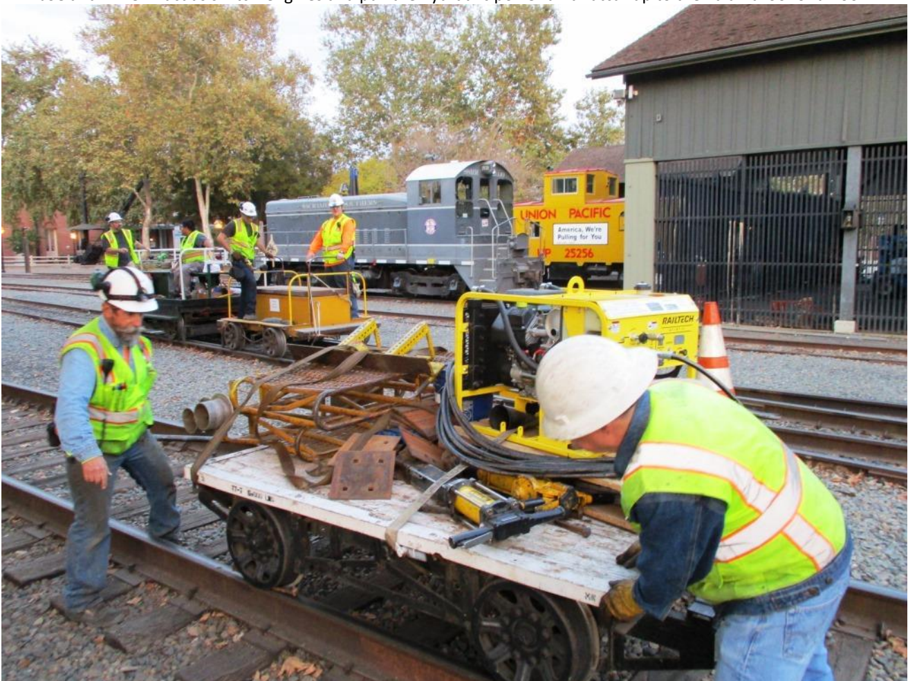
Joe and Mike H. spot the hydraulic power unit flat car while the rest of the Team bring the IHP bench car up the line
