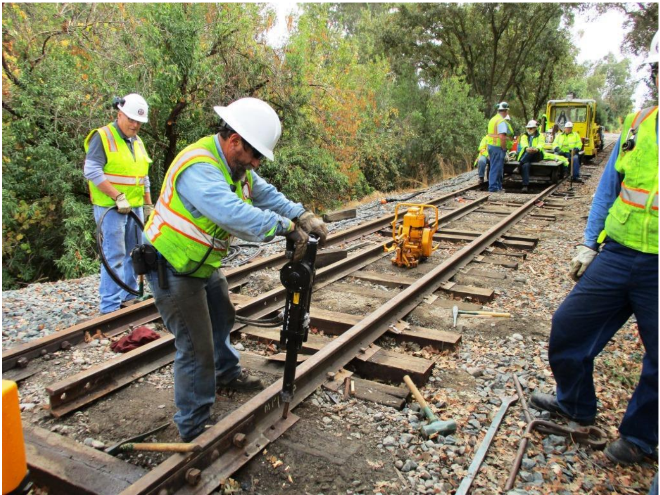
Joe's next on the new hydraulic spike-driver
