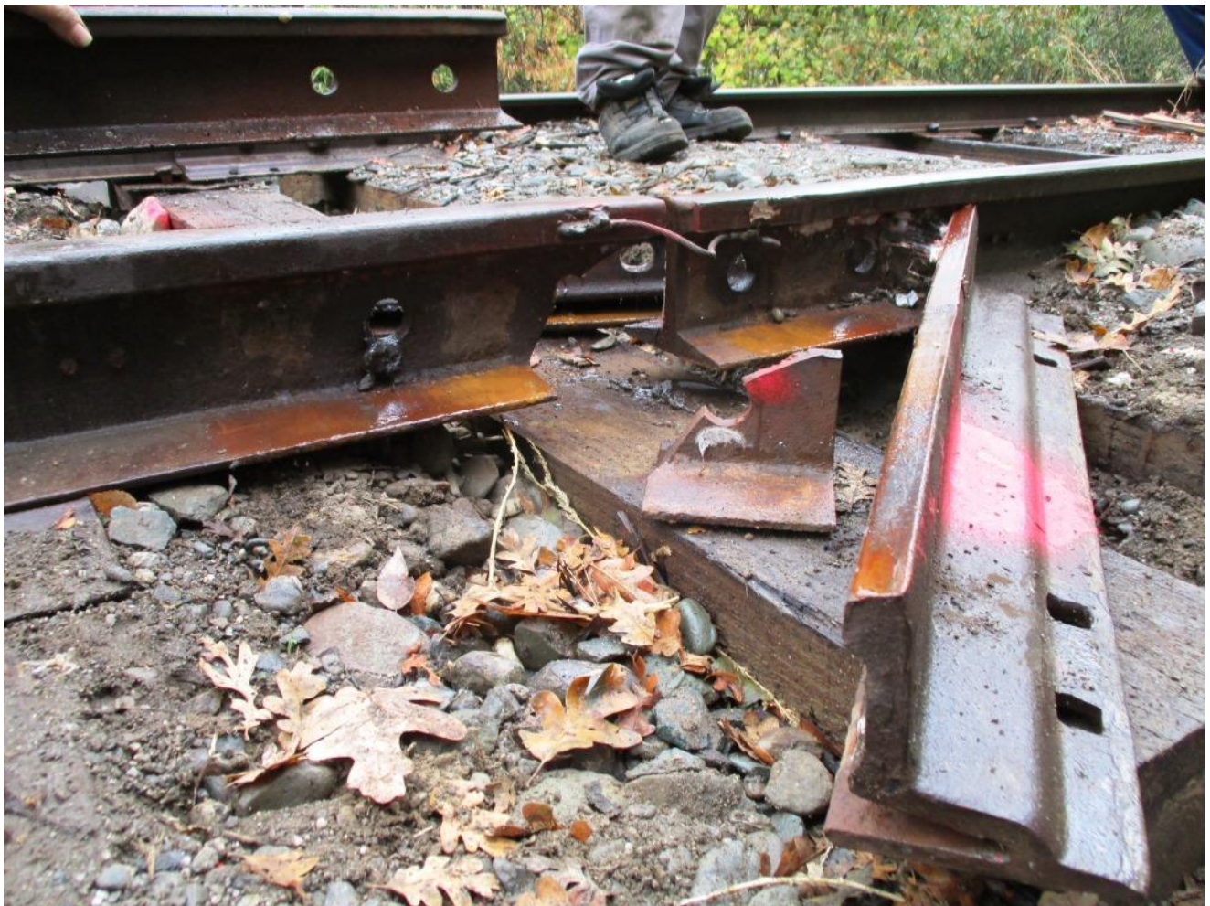
...To expose the busted rail
