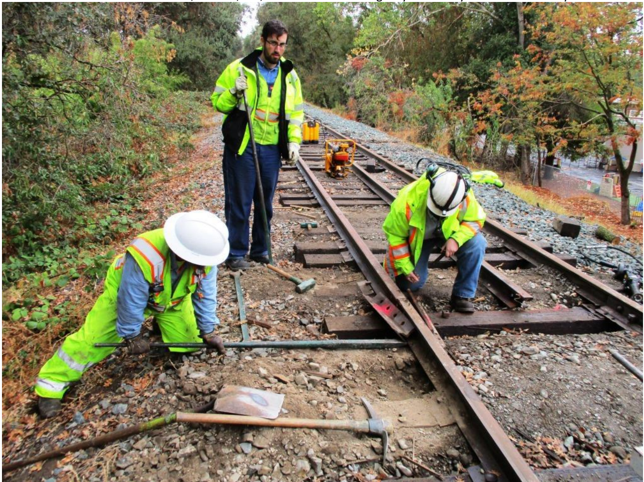
Joe uses a lining-bar to lever-up the rail to get level as Heather installs the joint-bars
