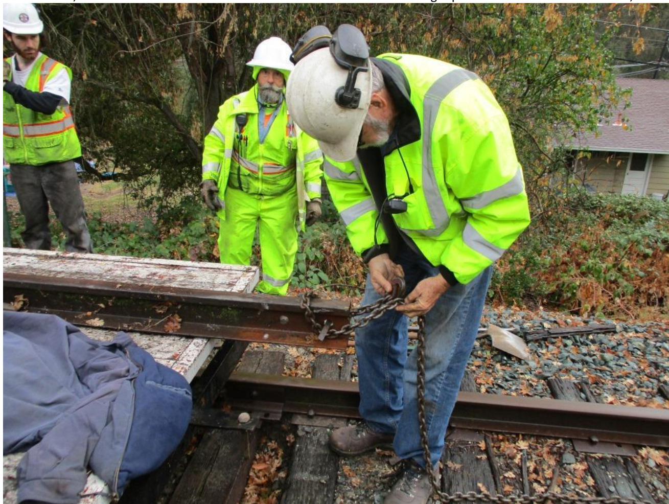
Alan attaches a chain to the new rail, the other end of which is anchored around the track
