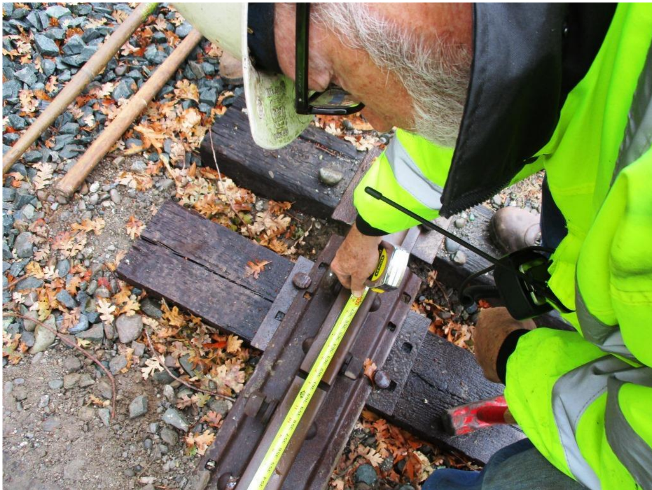
Measure twice, cut once: Alan double-checks the measurement on the rail being replaced. It's an odd size – 30-feet, one-inch
