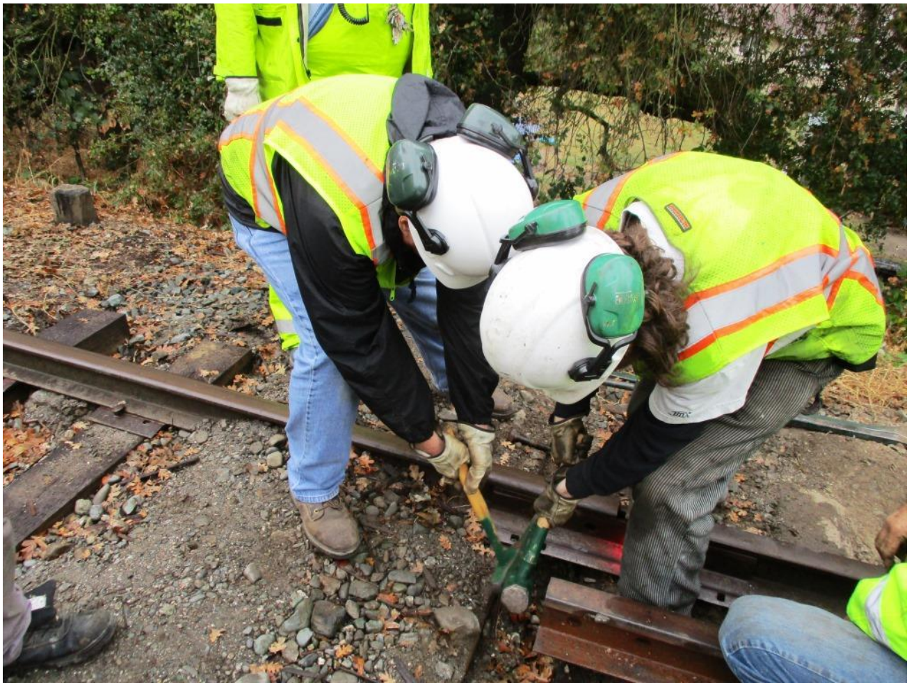
With the nuts removed, Bill and Matt use a track-punch to punch the bolt out of the joint
