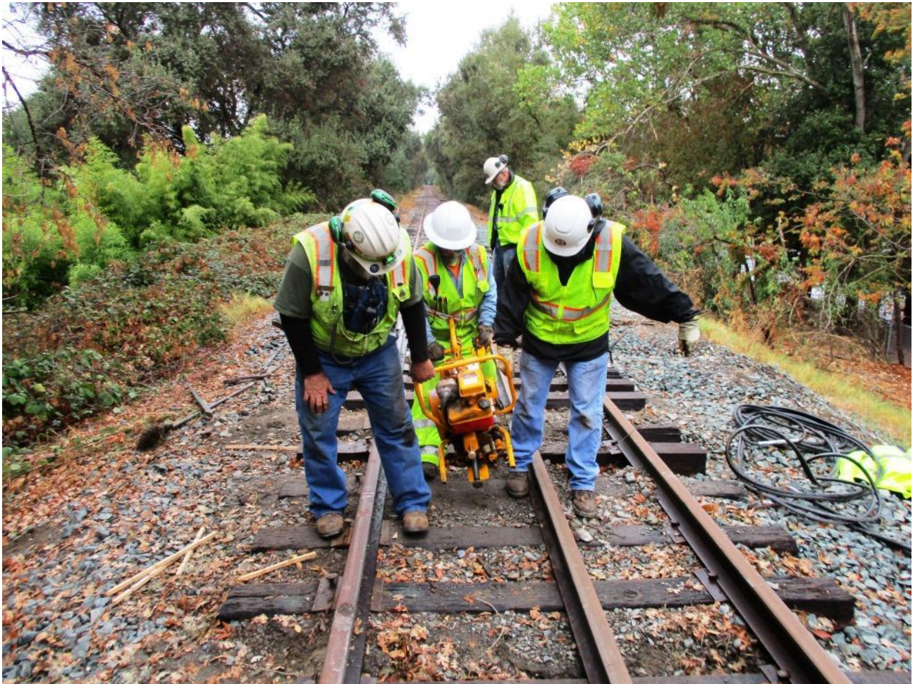
With the holes drilled, Mike F., Joe, and Bill move the ungainly and heavy drill out of the way
