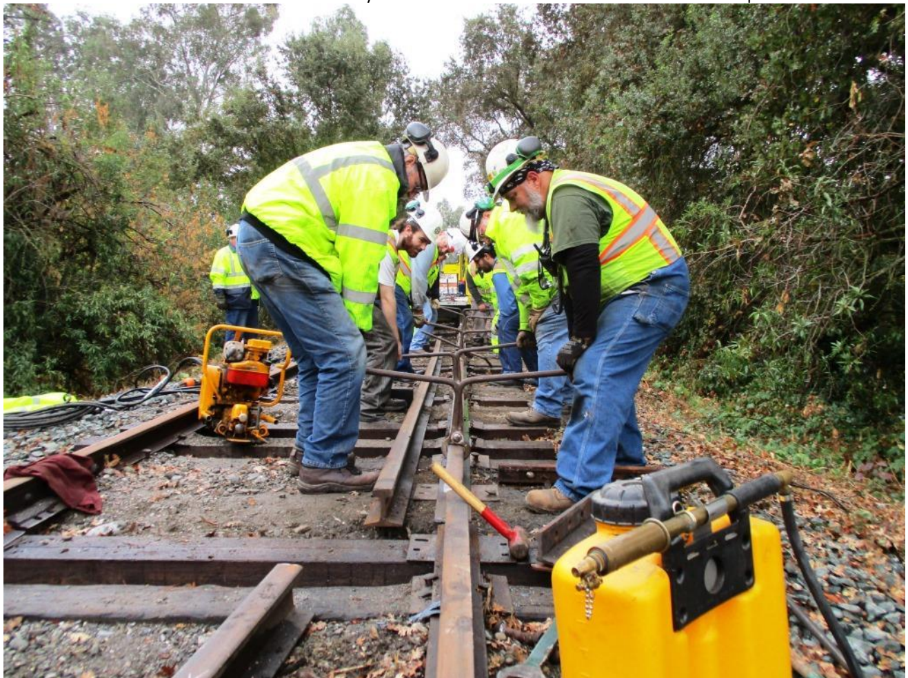
With the rail cut, the Team uses two-man rail-tongs to lift the new rail over the old and position it on the tie-plates
