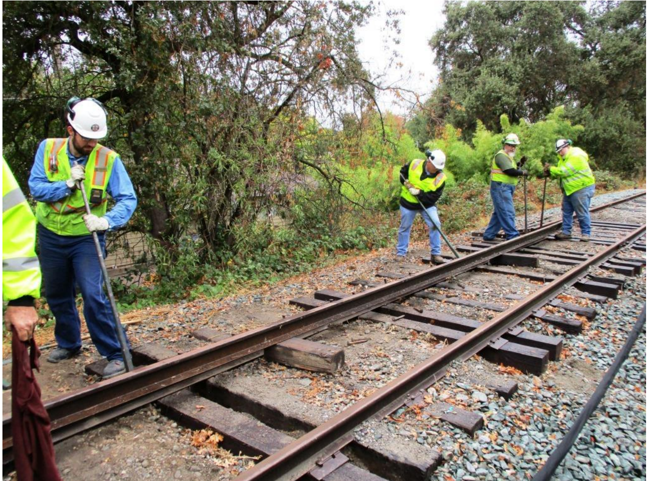
Weston, Bill, Mike F., and Frank demonstrate a little Gandy-Dancing as they use lining-bars to shove the old rail out of position
