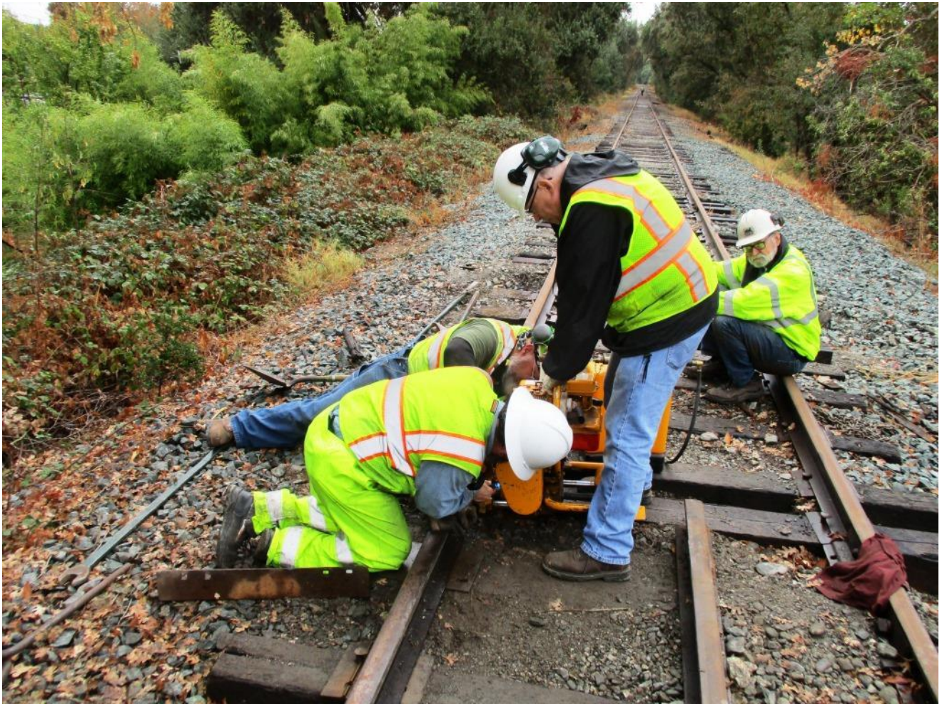
Mike F., Joe, and Bill position the rail-drill to cut new bolt-holes
