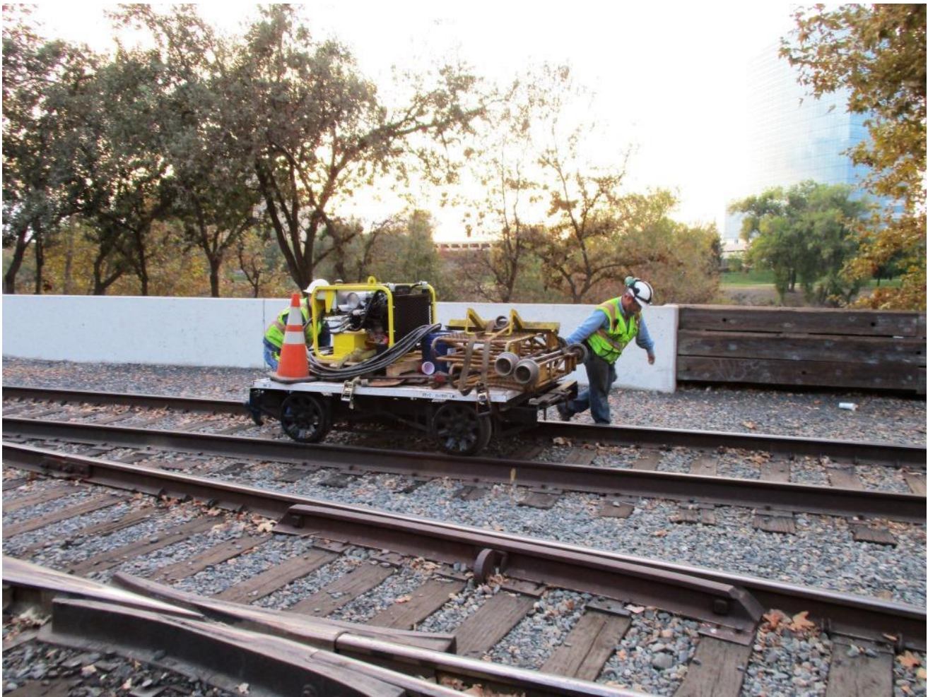
Joe and Mike H. act as switch-engines and pull the hydraulic power unit flatcar up to the Kalamazoo for a hook
